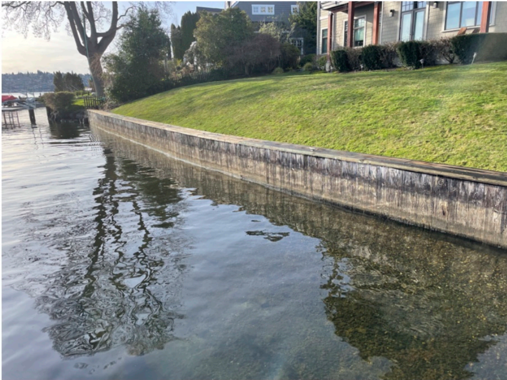
Photo 1 - Existing shoreline looking south
