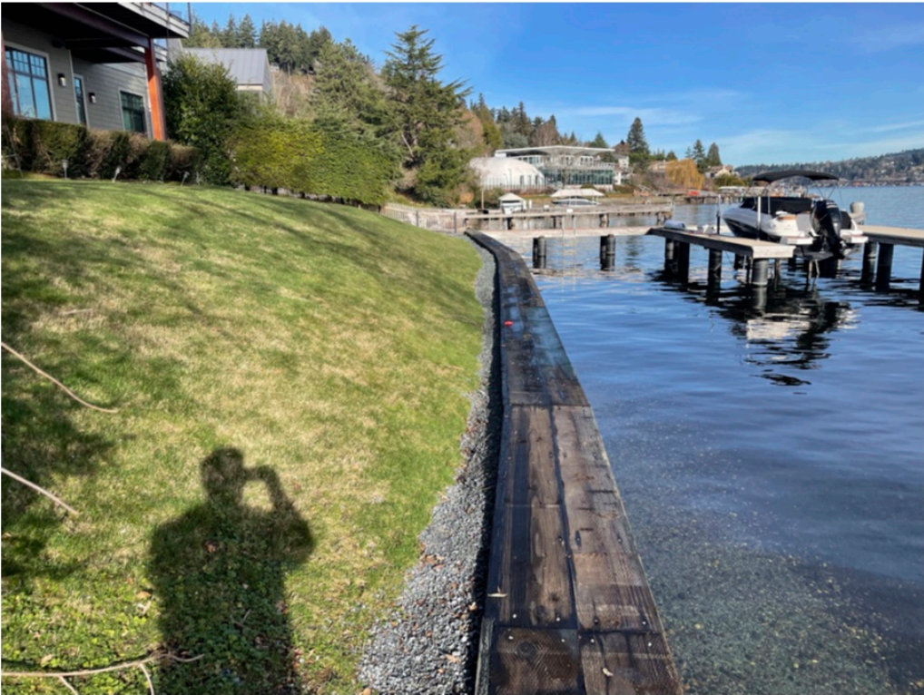
Photo 5 - Shoreline looking north along bulkhead.
